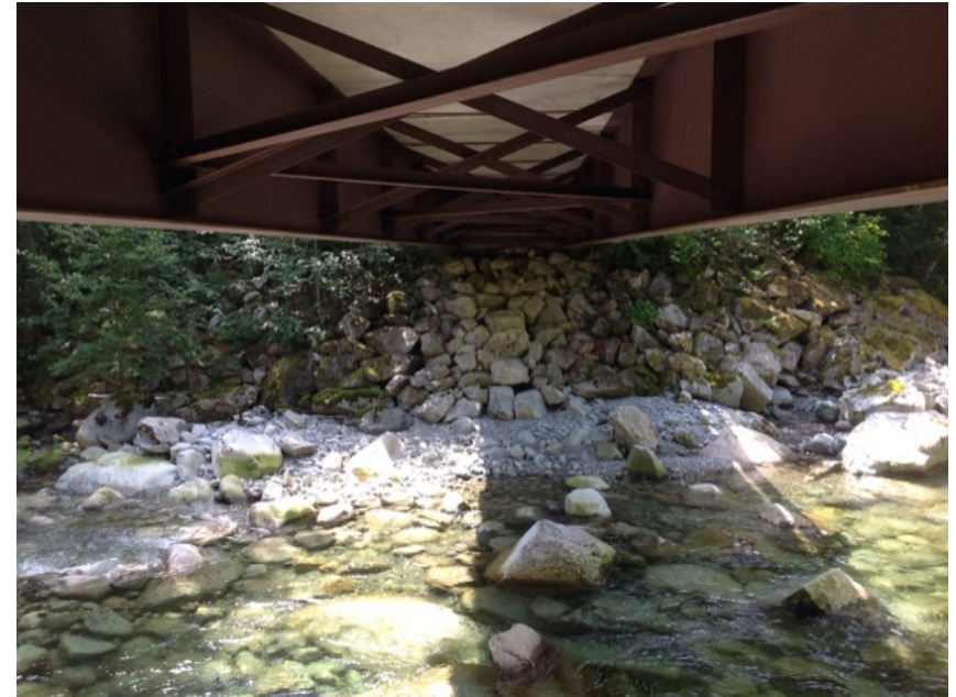
Right Bank Abutment when facing downstream
