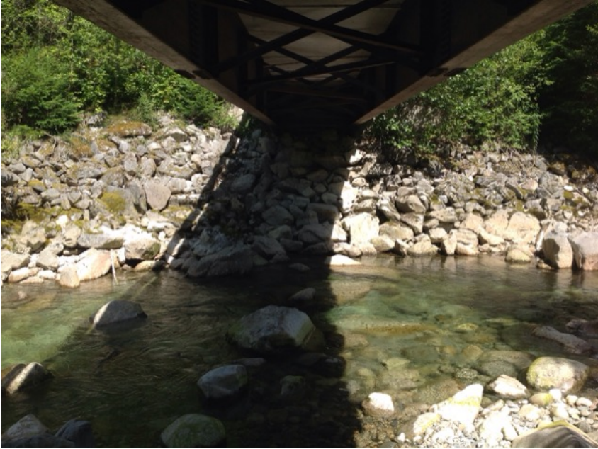
Left Bank Abutment when facing downstream
