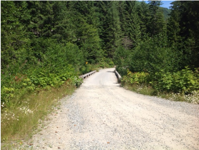
Approach from Right Bank when facing downstream
