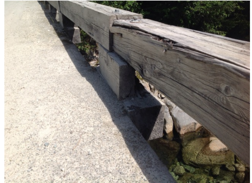
guardrail/riser condition
